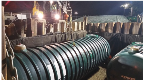
Left: Fuel tank installation Right: New float installed
