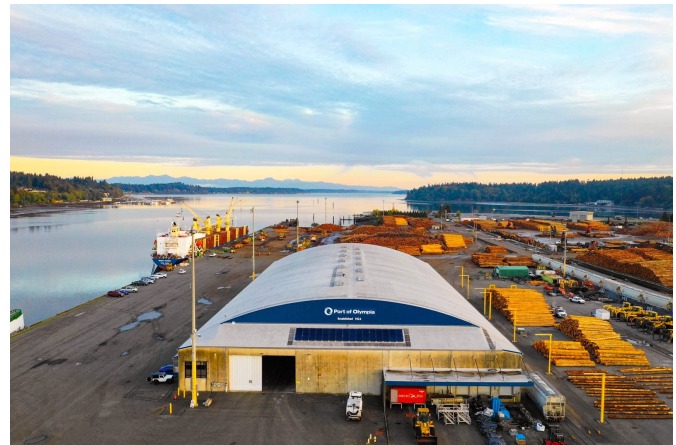
Marine Terminal warehouse and cargo yard.
