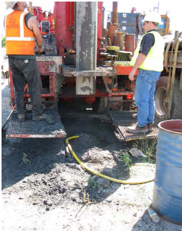
Photograph 2 – Hydrating the bentonite surface seal at AW-1.
