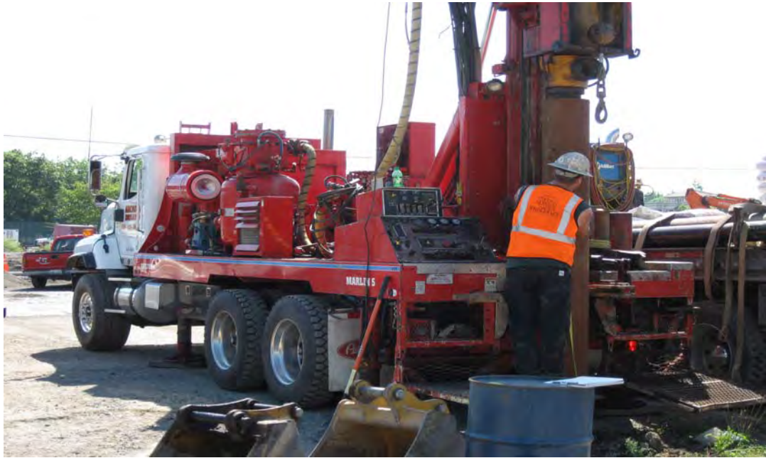
Photograph 1 – Overdrilling AW-1 prior to constructing the surface seal.
