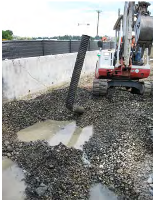
Photograph 4 – Corrugated drainage pipe in railroad bay (AW-2).
