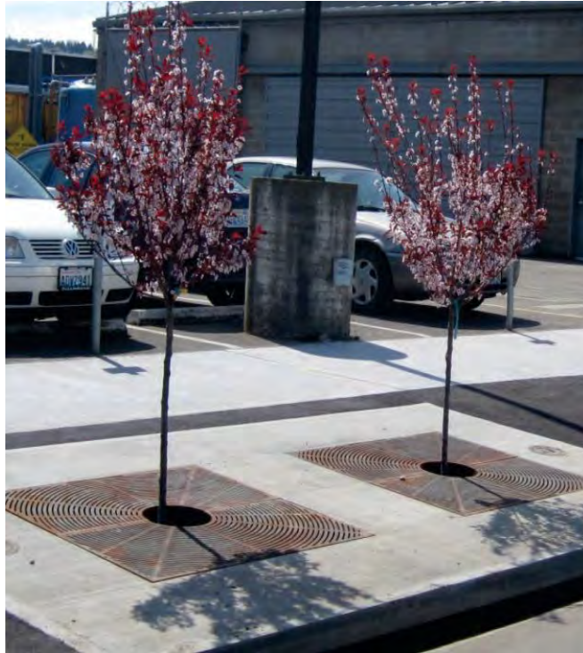
Figure 5 - Filterra® Bioretention System installed adjacent to sidewalk
