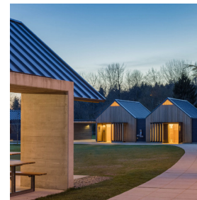
Juanita Beach Park Bathhouse, Kirkland, WA
