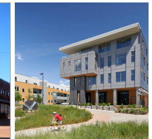
Commercial Mixed-Use Developments, Boulder, CO
