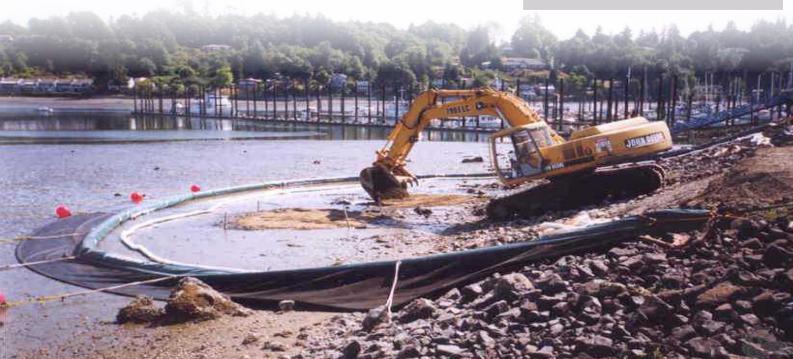
Sediment containment construction at Cascade Pole
